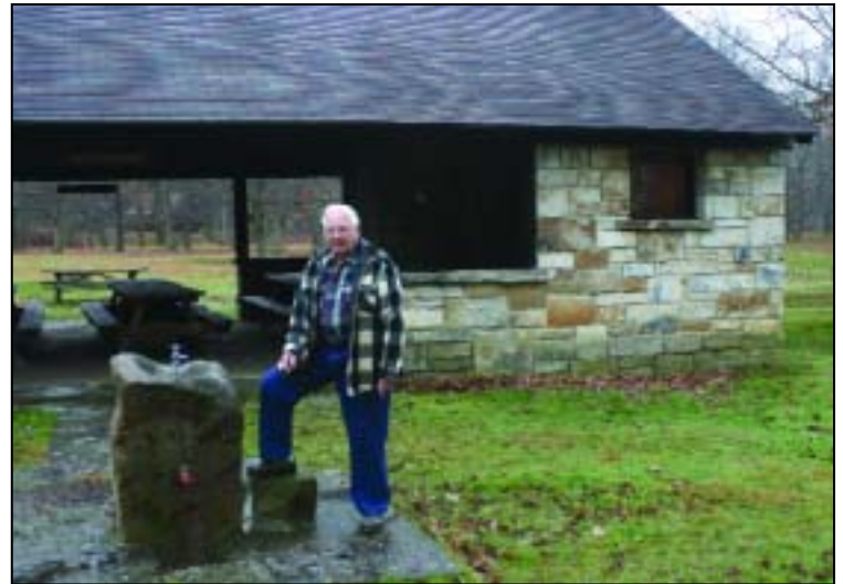
John Livengood helped build this pavilion back in the 1930's.
