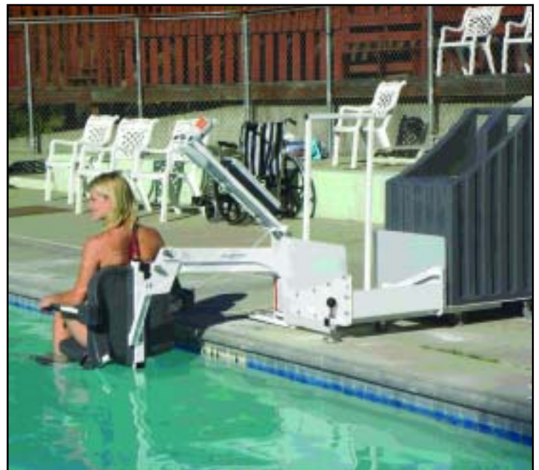
Keystone Funds were used to improve accessibility in state parks and forests such as adding a pool lift like the one shown in this photo.
